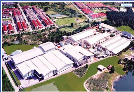
Factory premises in Ipoh, Perak, Malaysia
